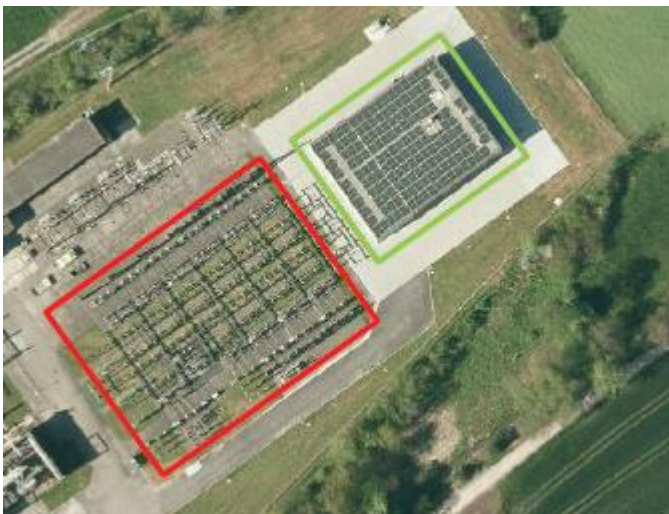
Location on the Altgass substation site
